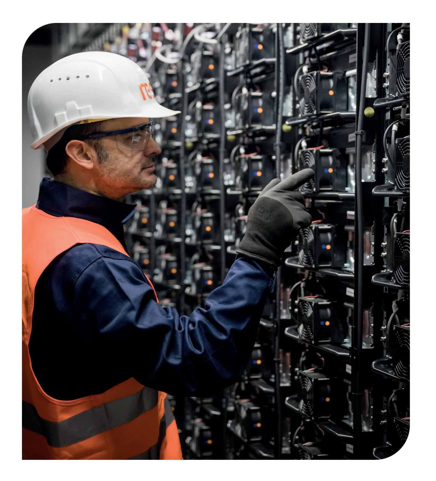
development is anticipated to be lithium iron phosphate (LFP). LFP has better stability against thermal runaway at higher temperatures compared to some other battery chemistries. All batteries must be tested and certified to an industry standard (UL9540A), demonstrating resistance to thermal runaway, and which ensures there is no likelihood of explosion, with any fire contained within the affected battery rack.
